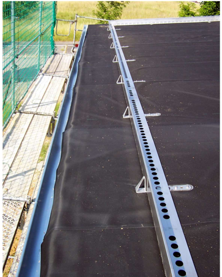
Shear barrier using ZinCo L-profile TRP80 or TRP140 in combination with ZinCo Shear bracket LF300
